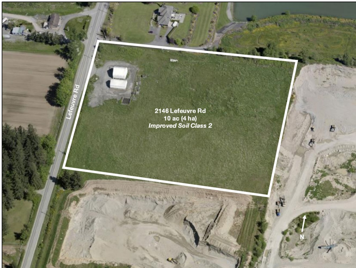
Figure 5 - 2146 Lefevre Road, Aerial Context (see Appendix A)
